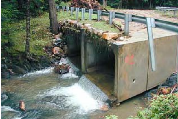
Double box culvert at Dingle Road (InterFluve Inc. photo)
