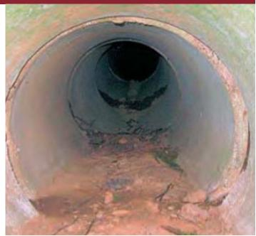
**Adequate**Minor separation of joints and seams up to 1", minor backfill infiltration.
