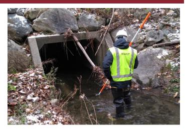
Observe the condition of the pavement or soil above the culvert and note any holes or cracks which could indicate a void underneath.
