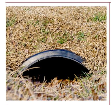
**Poor**Blockage is 30-75% of opening.
