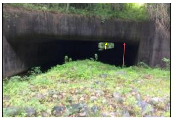
For this box culvert, the red arrow shows where to measure height above dry passage at the inlet – there is more clearance here than there is in the middle of the culvert immediately to the left, where rocks and sediment have mounded up. The yellow arrow shows where to measure height above dry passage at the
