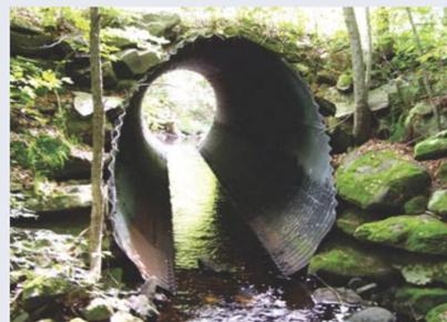
Shallow crossings have water depths too low for many organisms to move through them and may lack appropriate bed material. Crossings should have an open bottom or should be sunk into the streambed to allow for substrate and water depths that are similar to the surrounding stream.
