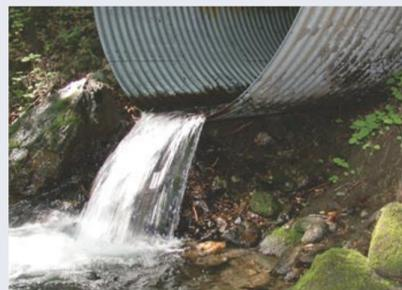
Perched crossings are above the level of the stream bottom at the downstream end. Perching can result from either improper installation or from years of downstream bed erosion. Crossings should be open-bottomed or sunk in the bed to prevent perching.
