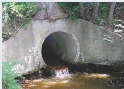
Undersized crossings restrict natural stream flow, particularly during floods, causing several problems, including scouring and erosion, high flow velocity, clogging, and ponding. Crossings should be large enough to pass fish, wildlife, and floods.
